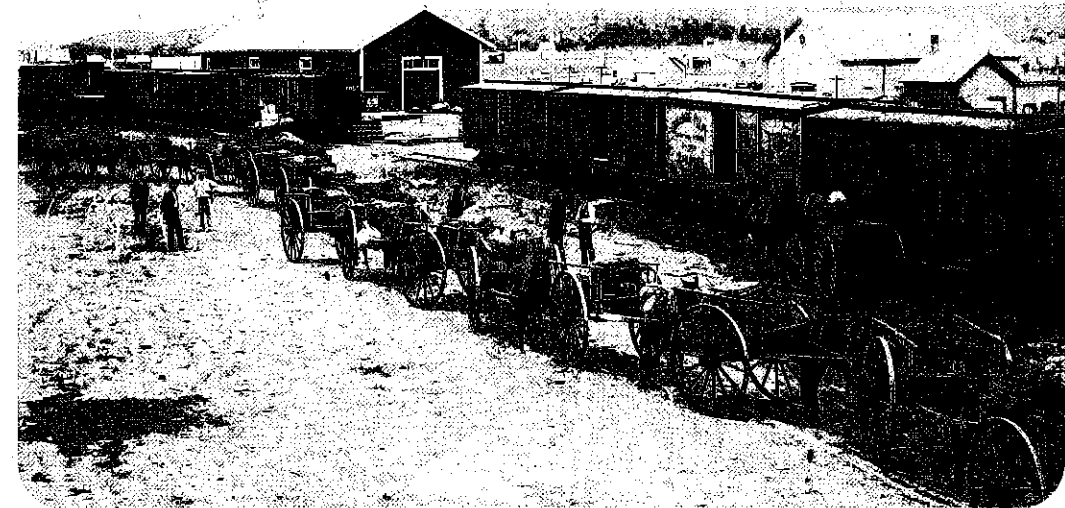
This 1888 photograph shows a line of Red River carts in Calgary. The Métis invented the Red River cart to transport goods, such as buffalo hides. It was easy to repair and its large, spoked wheels did not sink into the soft mud of the plains. The cart could also be used as a raft when the wheels were taken off. Grease was not used on the wheel axles because dirt would stick to the grease, so the wheels made squeaky sounds when they moved.
